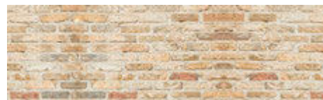
M24 Brick wall
