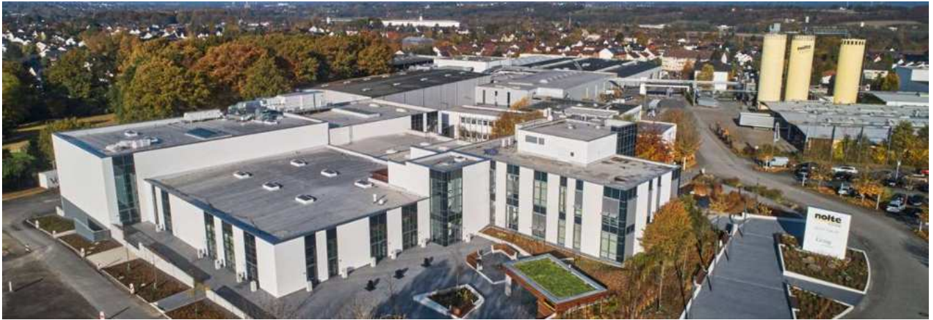
Nolte Küchen's operating base in Löhne, North Rhine Westphalia
