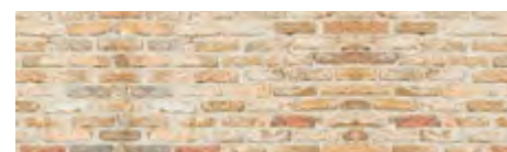
M24 Brick wall
